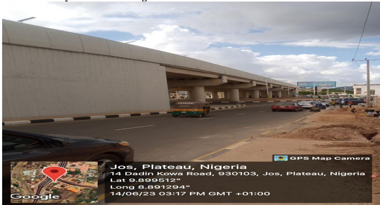
Plate 3: A newly constructed bridge on British-America Road
