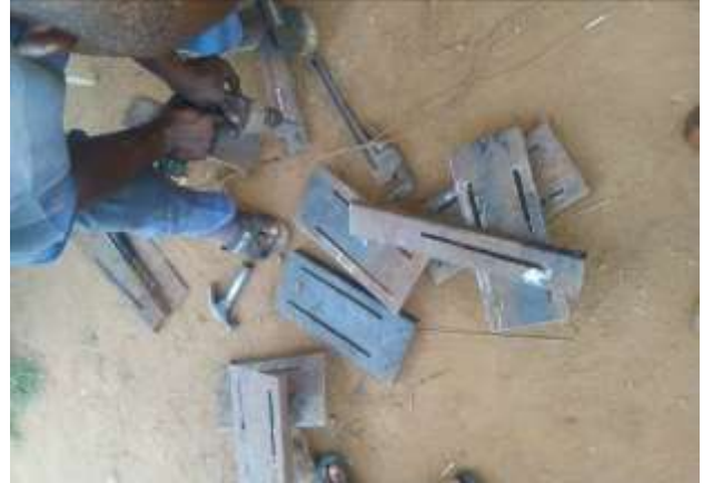
Plate 4.6: Drilling and smoothing of the metal plates before coupling
