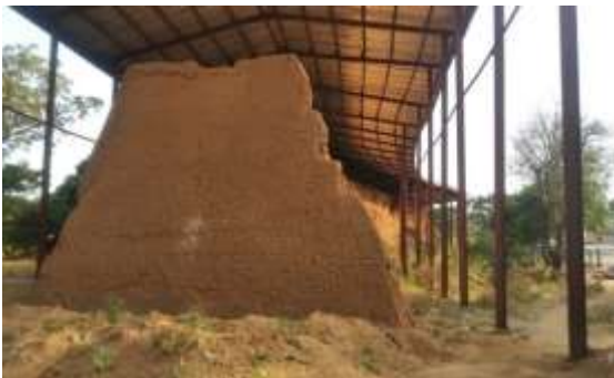
Figure 13: side view of Kano wall earth wall
