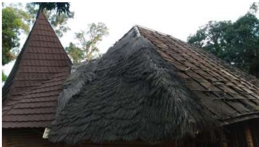
Figure 5: deteriorated thatch and bamboo poles sitting on aluminum and zinc corrugated sheets
