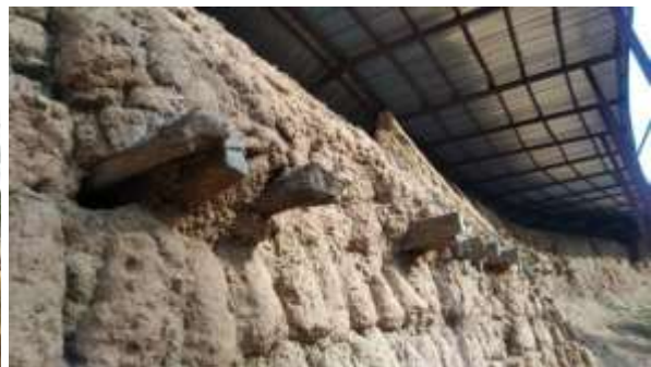
Figure 14: Exposed palm wood on earth wall
