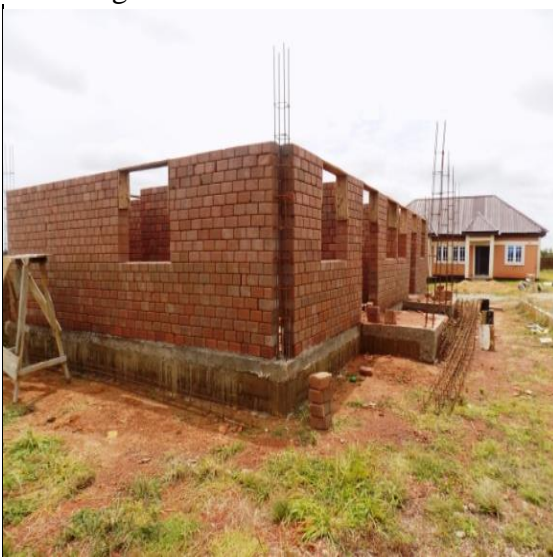
Plate v a & b: A house under construction using NBRI CEB technology in North-Central Nigeria
