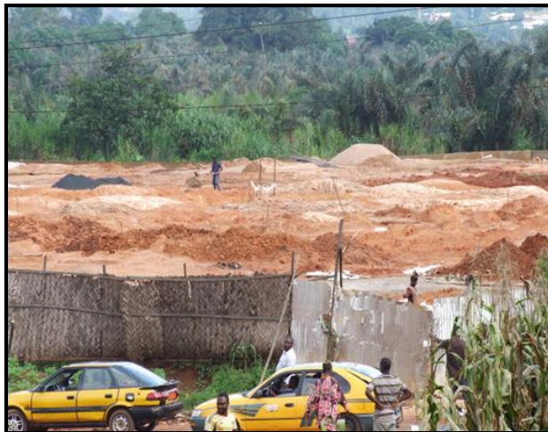
Photo 1: the land reclamation site
